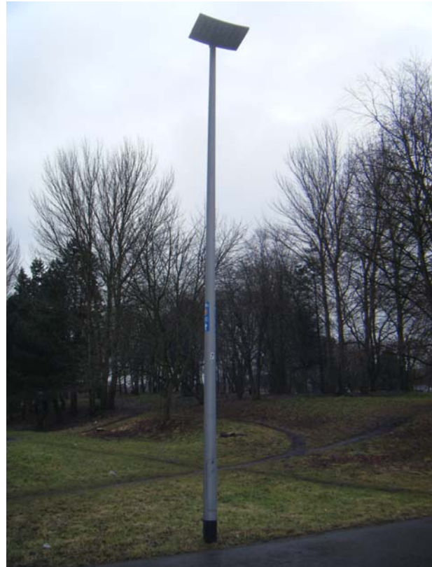
Steel Column with WRTL STELLA Luminaire
