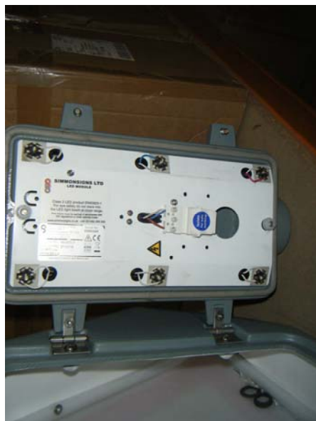
Retrofit LED Gear Tray for Sign Unit
